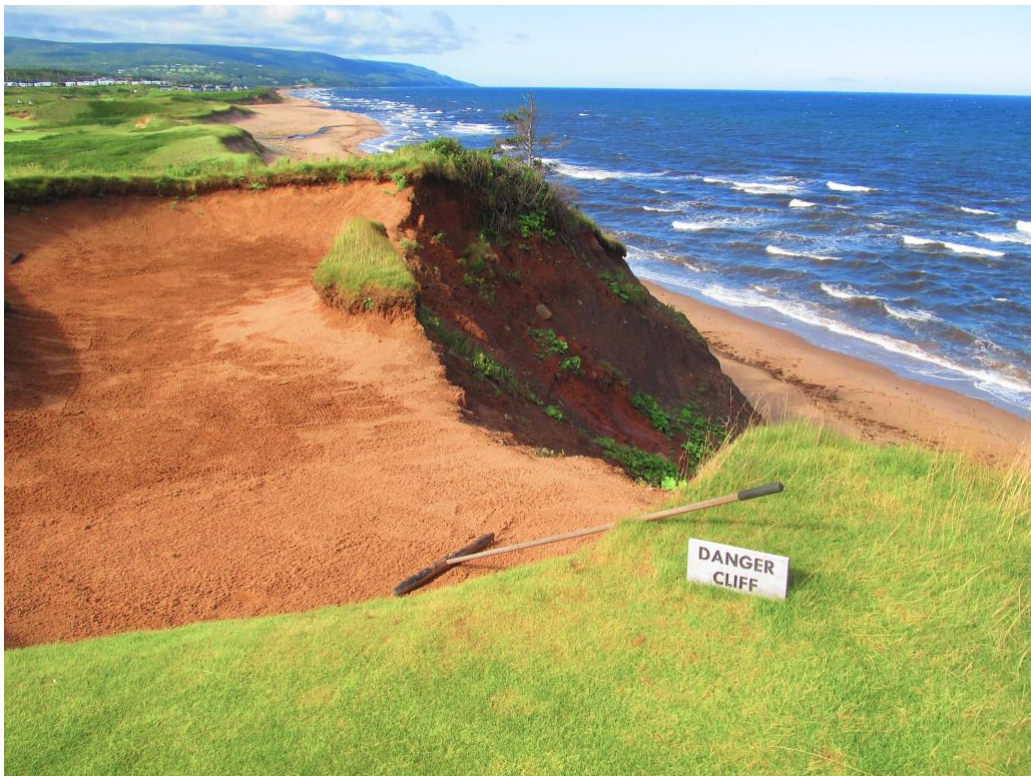
Dangerous Bunker Cabot Cliffs
